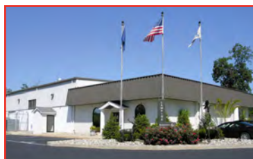
Biotech Research & Resource Center Pipersville, PA
